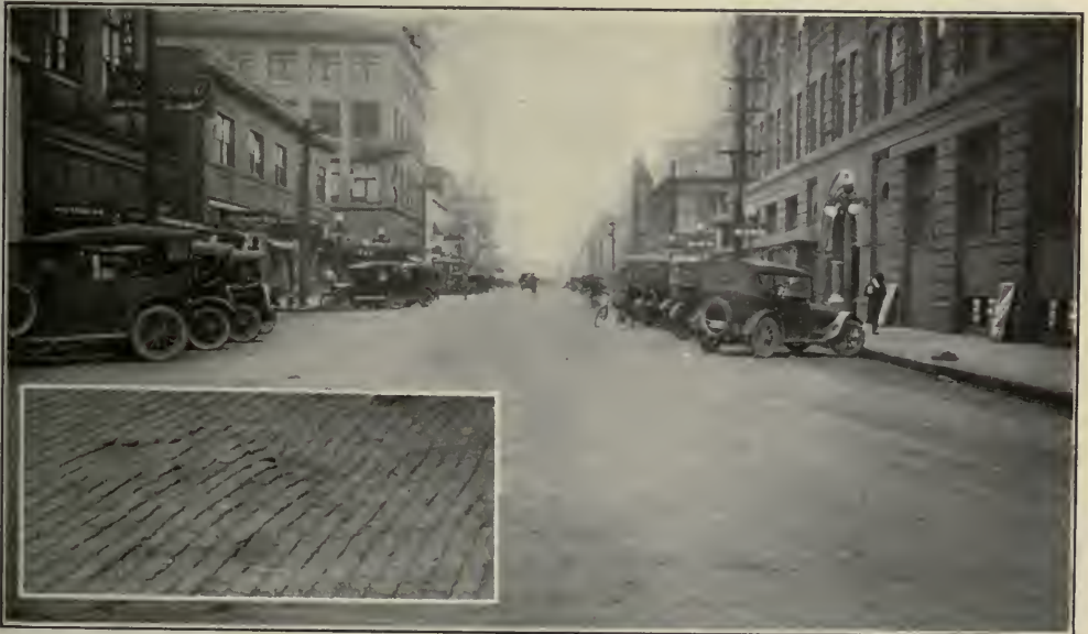
A STREET REPAVED WITH OLD BRICK—INSET SHOWS CONDITION BEFORE RELAYING
